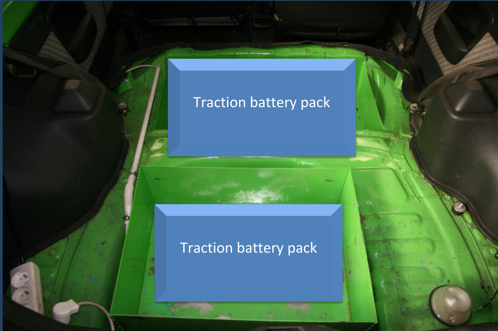
Pic.14. Battery area assembly under the rear seats.
